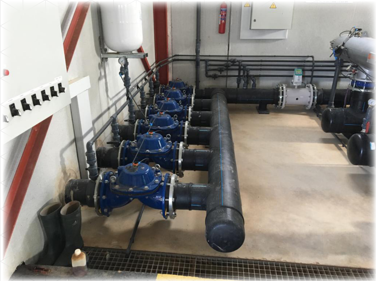
POLYETHYLENE OUTLET MANIFOLD WITH 6 VALVES HR10 8" Flange PN10
